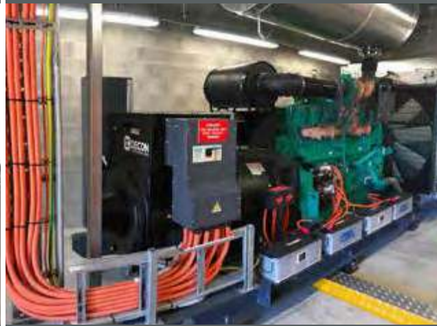
AUSTRALIA 2 X BASE FRAME 825/750 kVA
