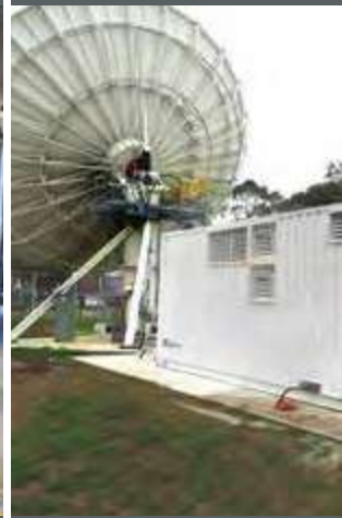
AUSTRALIA SATELLITE PLANT 2 X GENSETS IN CONTAINER 2
