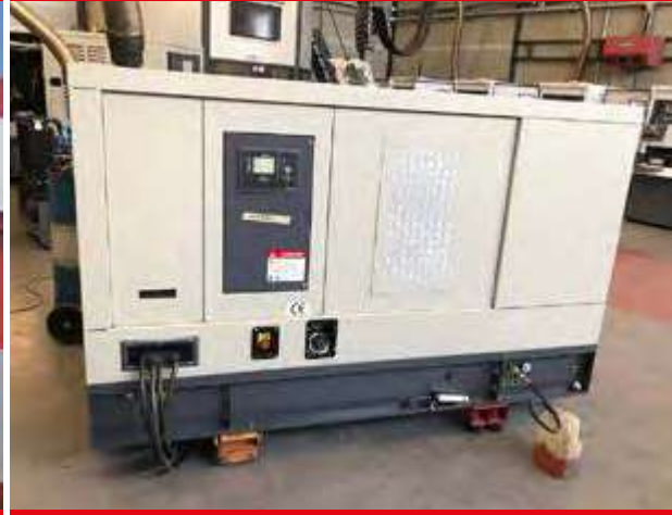
200 KVA VEHICLE FOR MILLS
