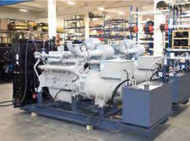
800 KVA WITH DOUBLE WALL TANKS 1000 LTS
