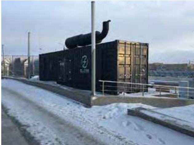
KAZAKHSTAN GENSET IN CONTAINER 40'1880/1700 kVA
