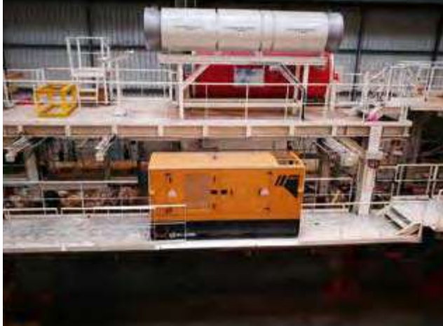
FRANCE - UNDERGROUND WORK 4 X GENSET 225/205 kVA
